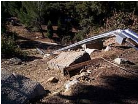
Steep grade and environmental conditions Required insulated pipe and special design features.
