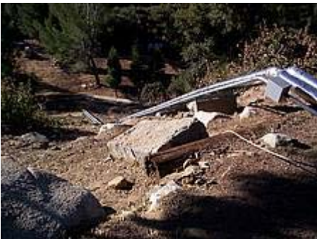
Steep grade and environmental conditions Required insulated pipe and special design features.
