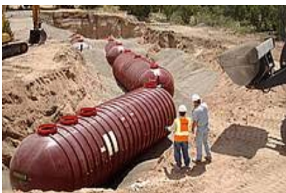
Installation of four 20,000 Gallon Tanks ( Primary And Recirc)
