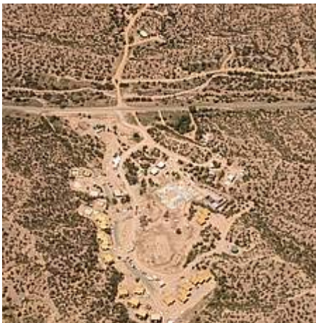
Aerial view of the Rancho Encantado Resort during renovation
