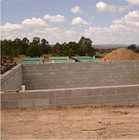
Construction of the outer perimeter of the Upflow Nitrogen Reduction Filter.
