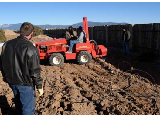
IWS preparing to install drip irrigation with a Vibratory plow.
