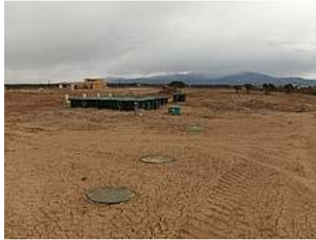
Construction of treatment system nears completion
