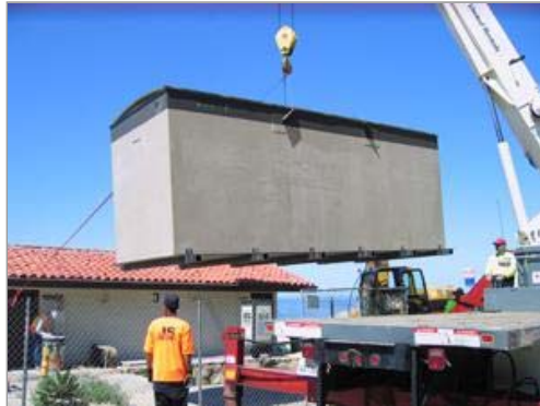
Juan Ramirez of JS Innovative Systems helps a crane operator from United Rentals maneuvering a 6,500-pound AdvanTex AX-MAX module from the delivery truck. (Photos courtesy of BioSolutions Inc.)
