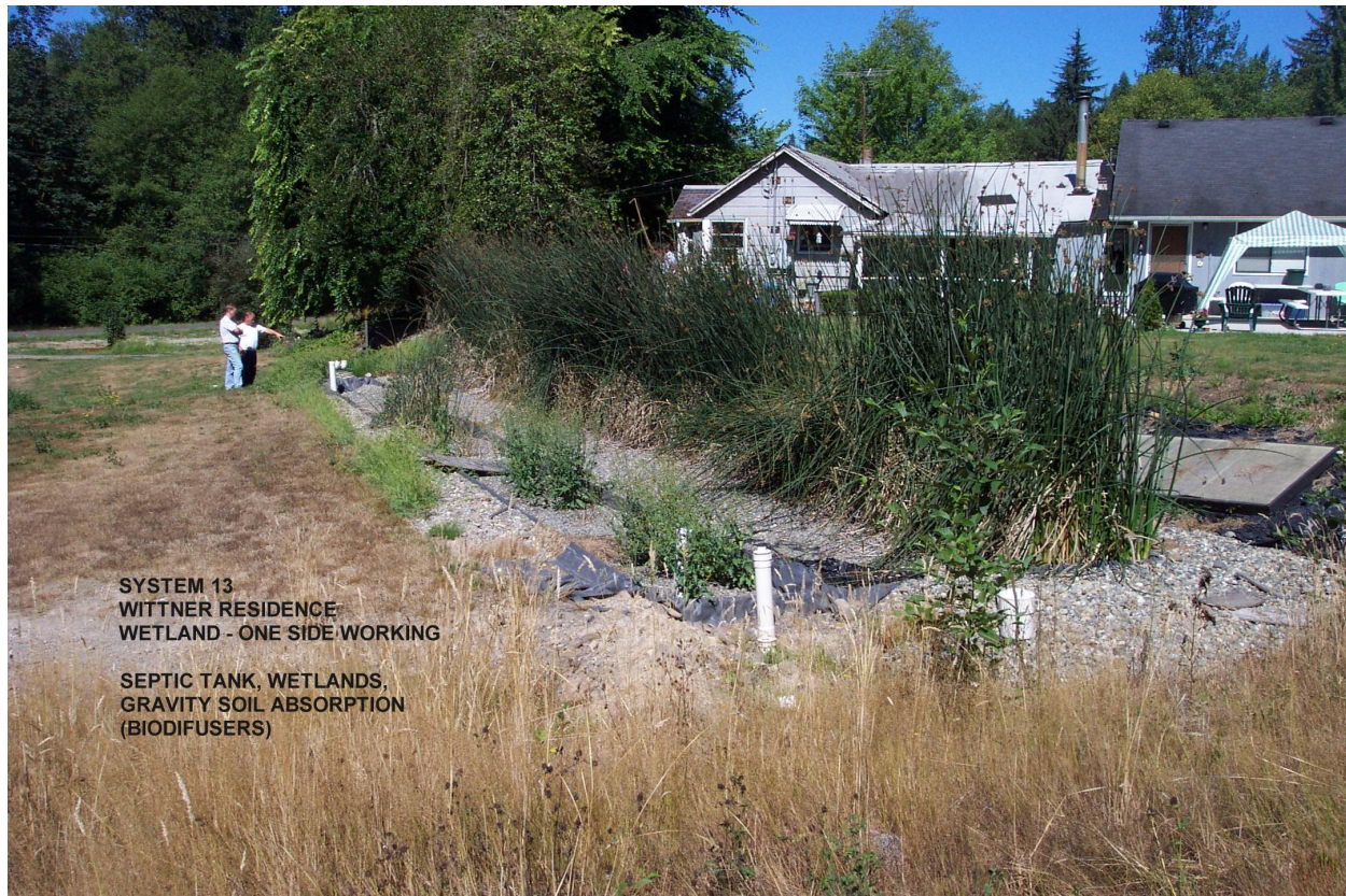
Figure 2: Five sq. m. wetland treating septic tank effluent from a single family home.
